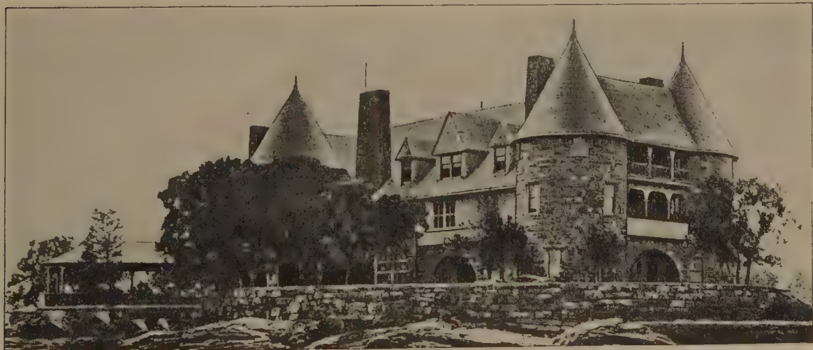
391 McKim, Mead and White, architects; © Architectural Book Publishing Co.
